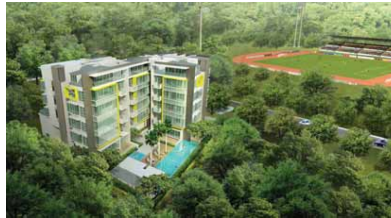
WEMBLY RESIDENCES - Yio Chu Kang Road (Apartment)
